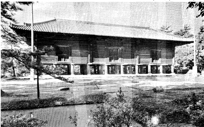
Shōsō-in of the Tōdai-ji, Nara, built c. 1752 in the azekura-zukuri style, Late Nara period. The only extant example of a shōsō , or repository, built to hold a temple's most treasured objects.
